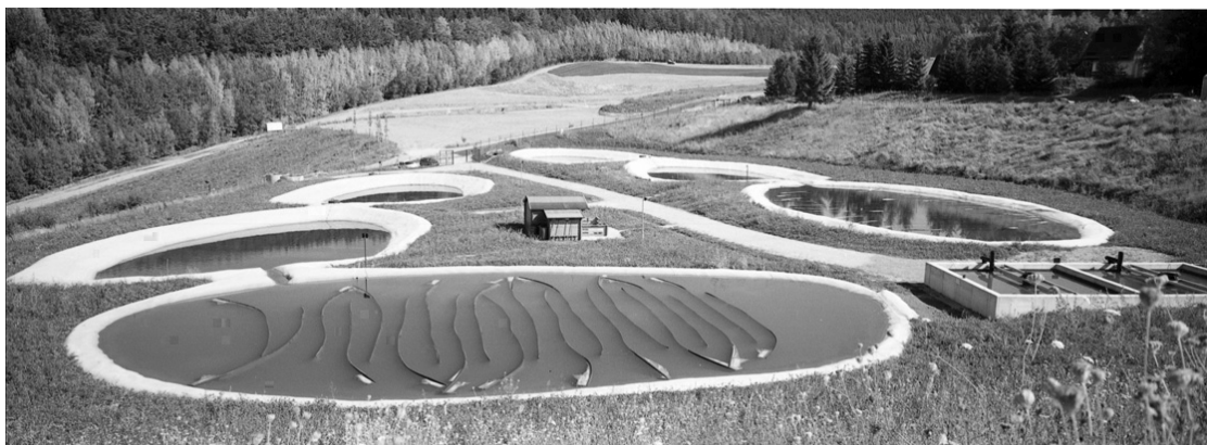
Figure 7: Photograph of the constructed wetland at Poehla, Autumn 2004
