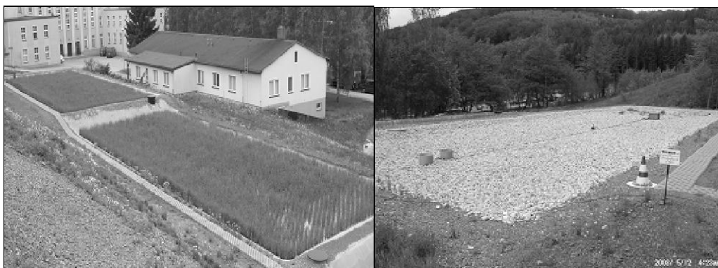
Figure 8: Experimental multi-cell wetland at WISMUT's Schlema mine site (left: plant cells, right: microbiological cell with gravel bed)
